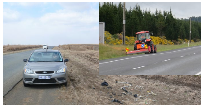
Figure 8: Road reserves that are disked, create a more effective fire belt
